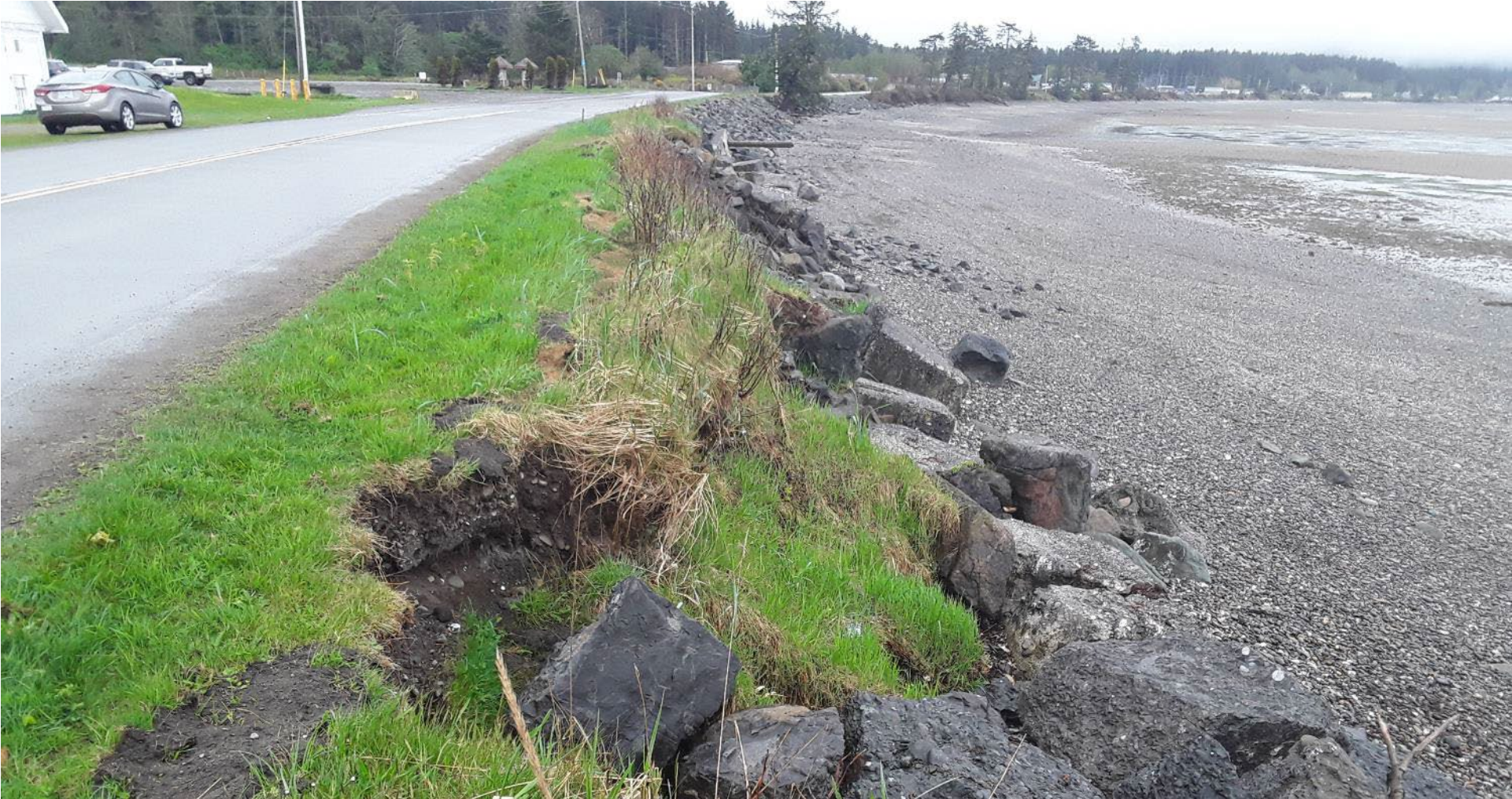
Damaged shoreline rock protection structure.
