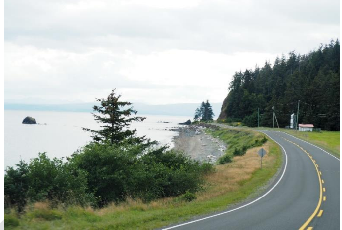
Figure 4: Highway 16 - Potential Area of Erosion Concern
