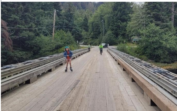
Figure 8: Towhill Road - Sangan Bridge
