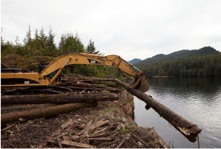
An excavator is used to haul the debris from the collection site up on to the bench for dewatering
